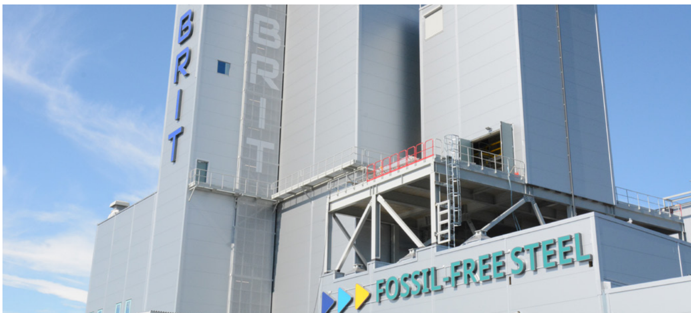
HYBRIT pilot plant (Credit: SSAB/Åsa Bäcklin)
