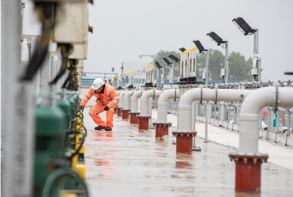
Figure 4: Deephams Sewage Treatment Works
