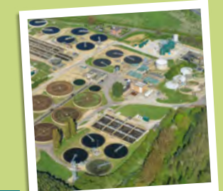
Bedford Water Recycling Centre
